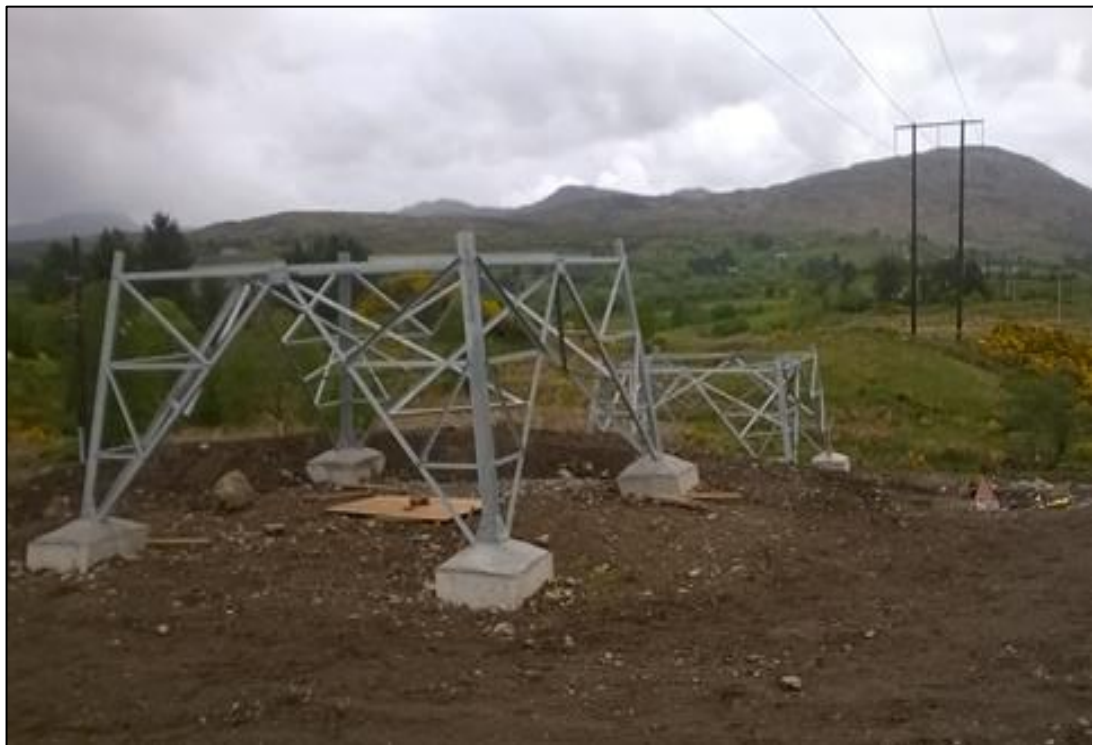
Plate 4-10 Steel lattice tower foundation complete (example image)
