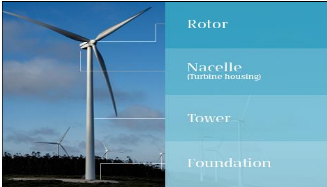
Plate 4-1 Wind Turbine Components
