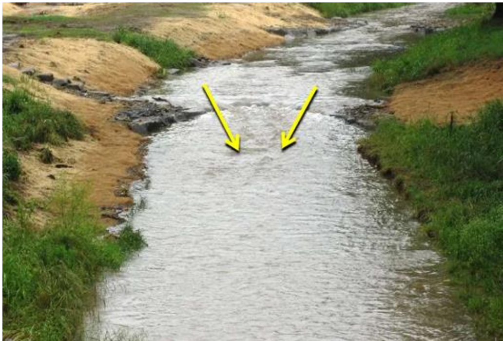
Plate 4-4 Example of cross vane on a restored stream
