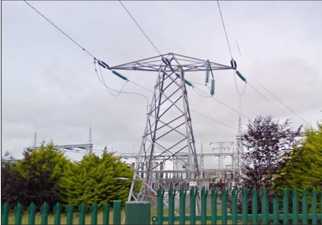
Plate 4-11 Completed End Mast Tower (example image)
