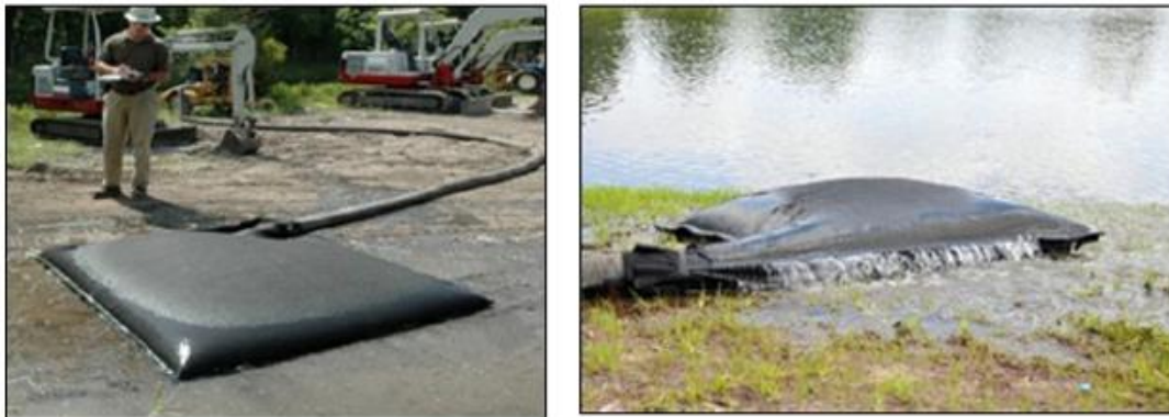
Plate 4-7 Silt Bag with water being pumped through.
