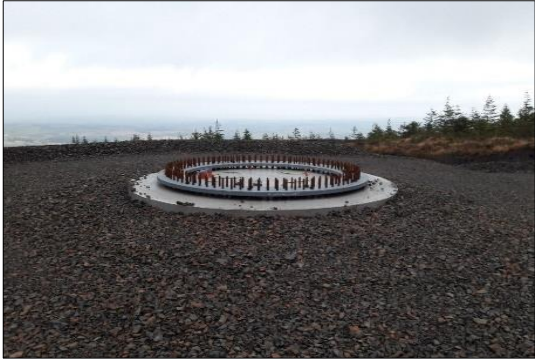
Plate 4-3 Finished Turbine Foundation
